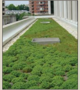
Green roofs are an example of sustainable design.
