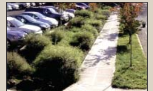
Green streets better accommodate stormwater management techniques, such as curb-cuts to infiltration basins and rainwater gardens.
