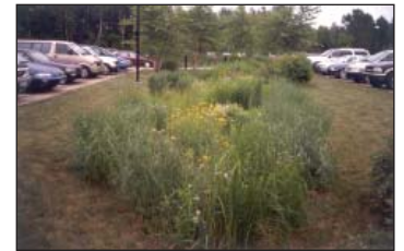
Rainwater gardens are one of many environmentally sensitive design elements to encourage a healthy community.
