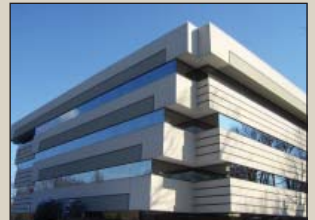
SoBo Tech Center
