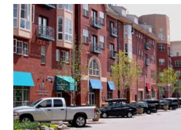
Angled parking serves ground level retail uses
