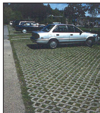
Pervious pavement for parking areas..
