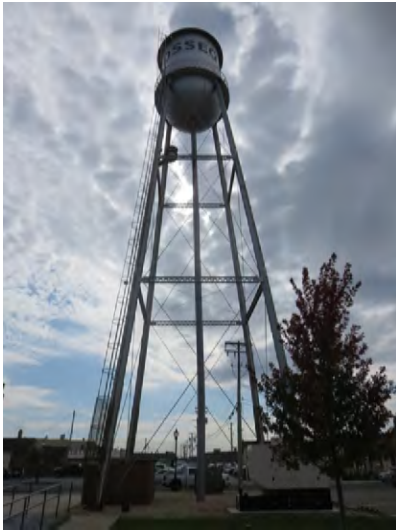
Tower, looking south.
