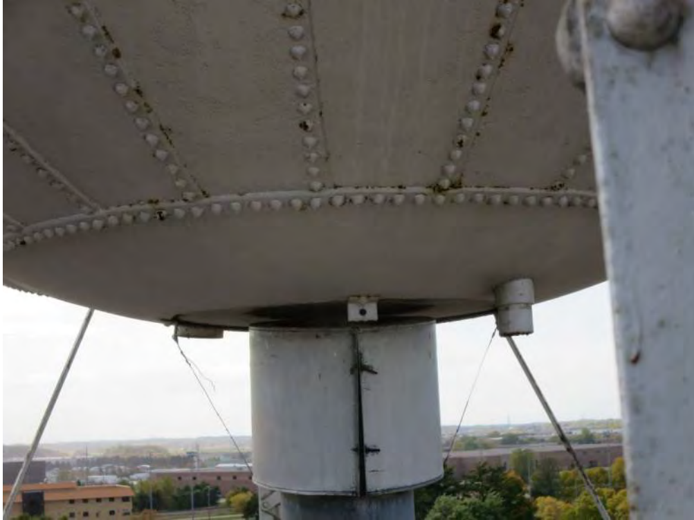
Photo 14 - Base of tank
