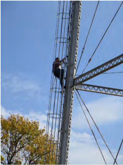
Ladder and cage at northeast leg of the tower.
