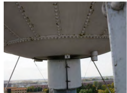
Expansion joint between the riser and the tank.
