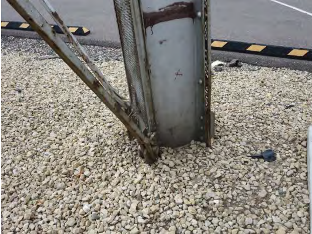
Photo 4 - Northwestern column base
