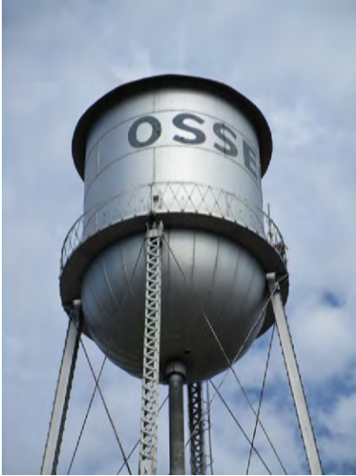
Osseo Water Tower tank, photograph looking northeast.
