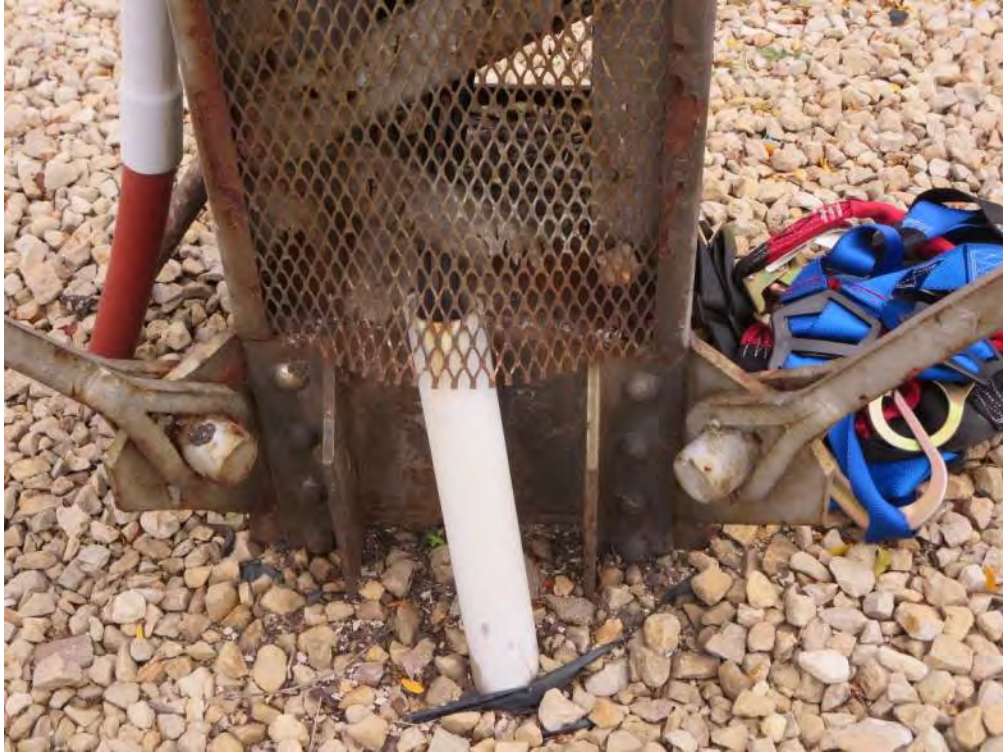
Photo 2 - Northeastern column base
