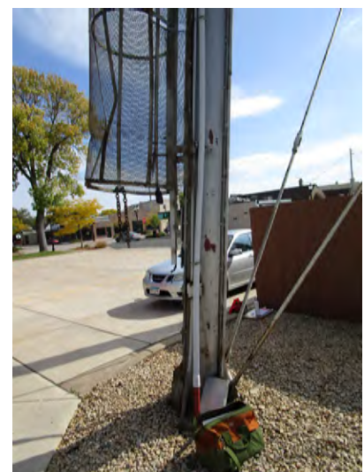
Bottom of ladder cage at northeast leg of tower.
