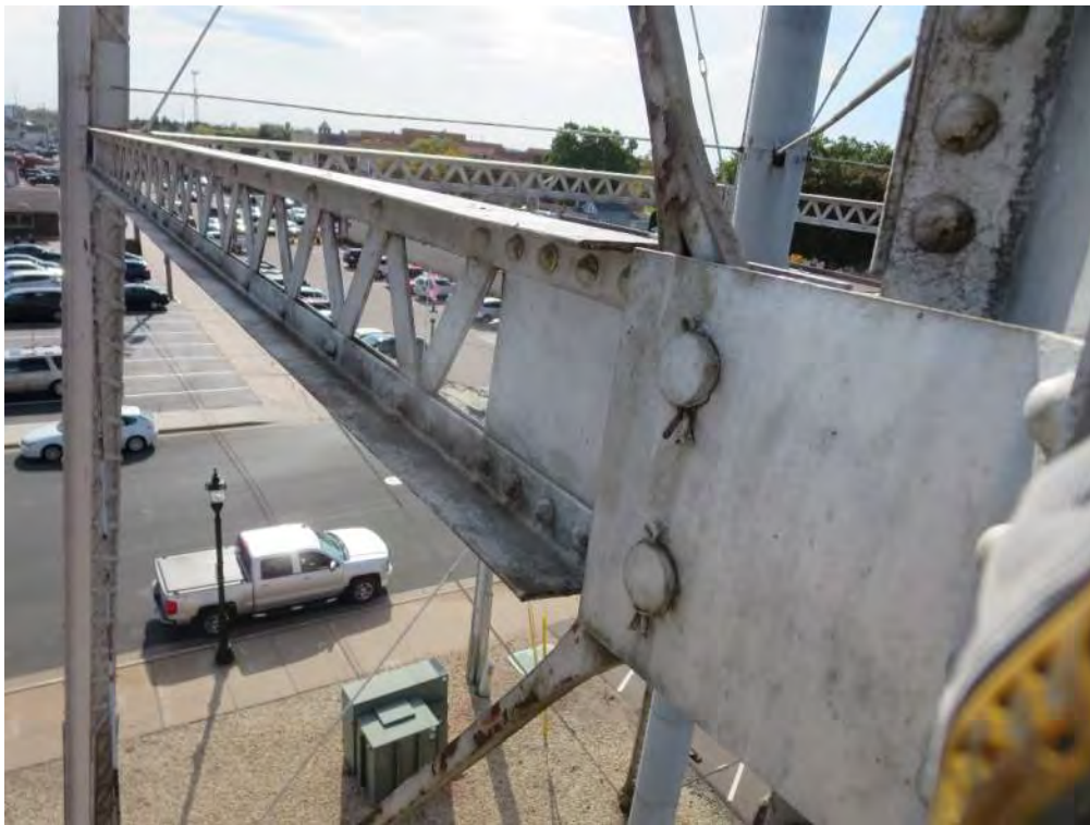
Photo 7 - Horizontal beam - note: cotter pins intact
