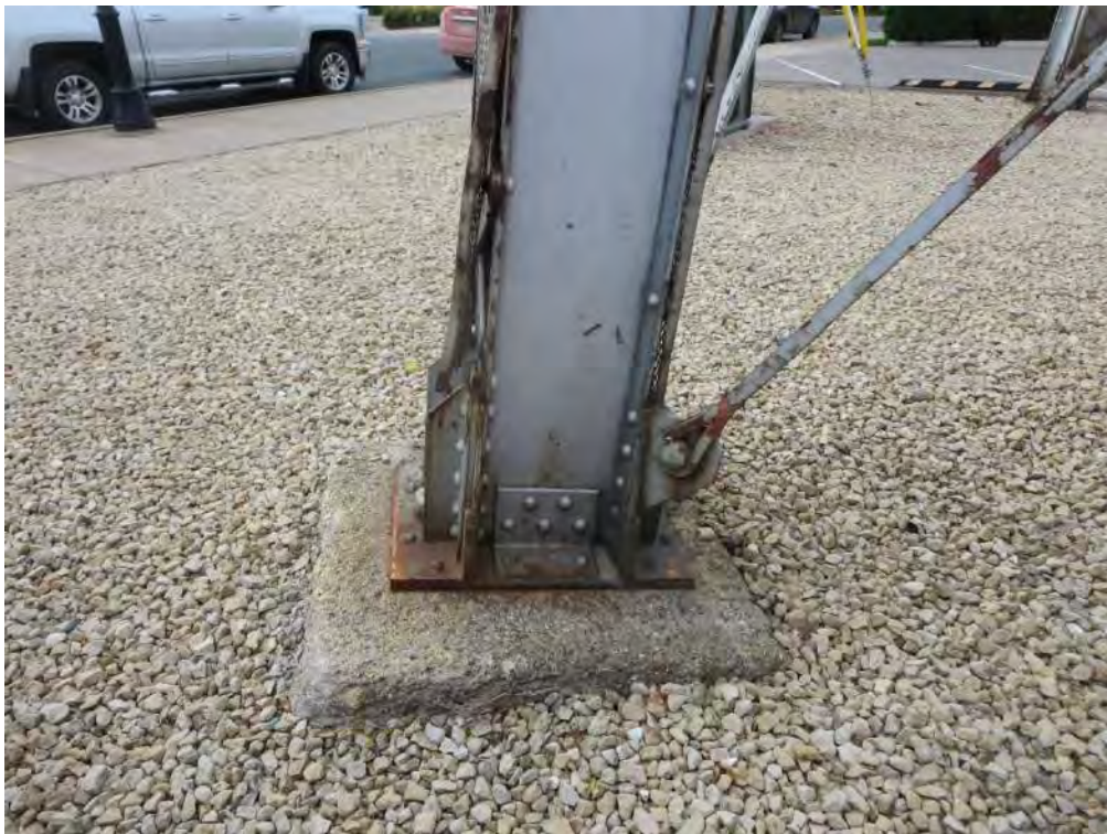
Photo 3- Southeastern column base
