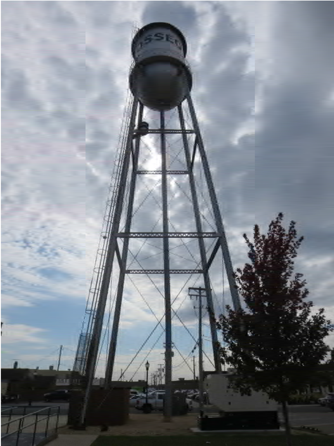
Photo 1 - Water Tower Overall, facing south
