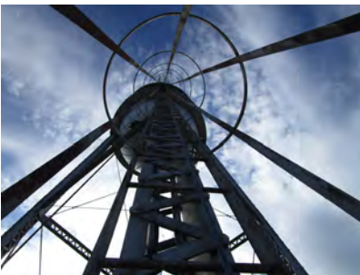
Photograph looking up from the inside of the ladder cage.
