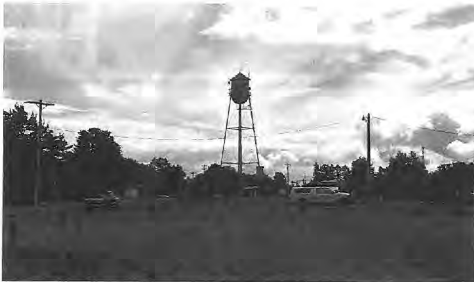
(SOURCE: AKAY Consulting, Floodwood, MN, September 2014)
