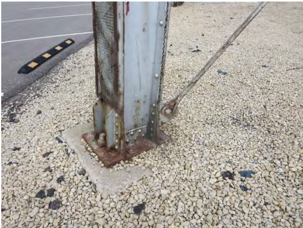
Photo 5 - Southwestern column base
