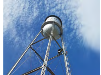
Photograph taken by the southeast leg of the tower.
