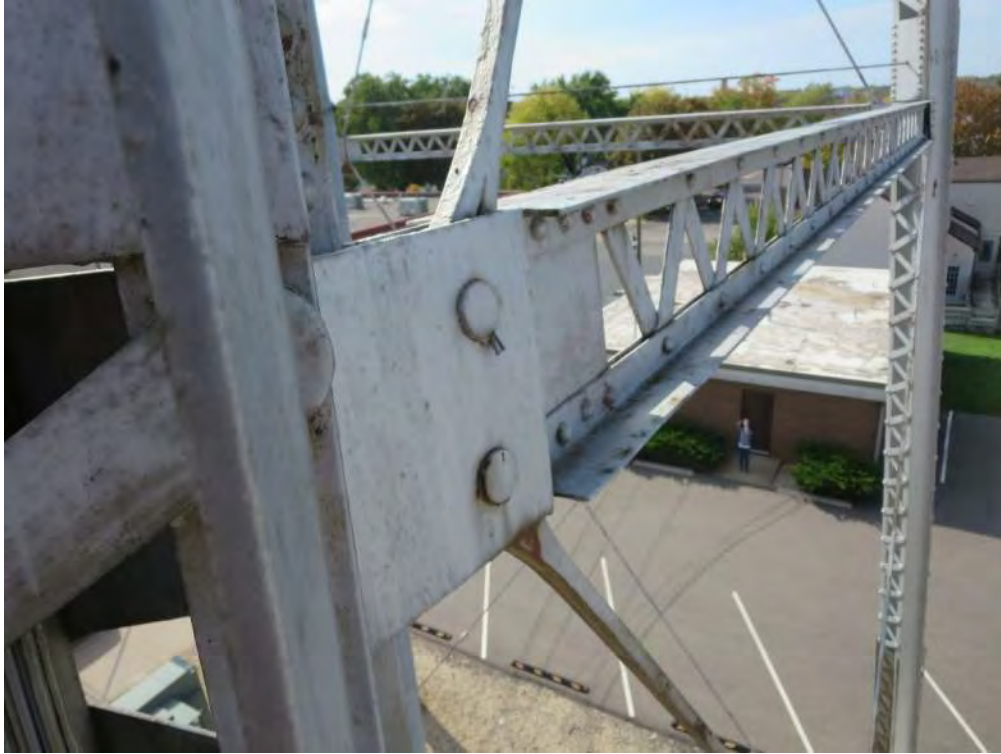
Photo 6 - Horizontal beam - note top cotter pin broken at top, bottom cotter pin missing
