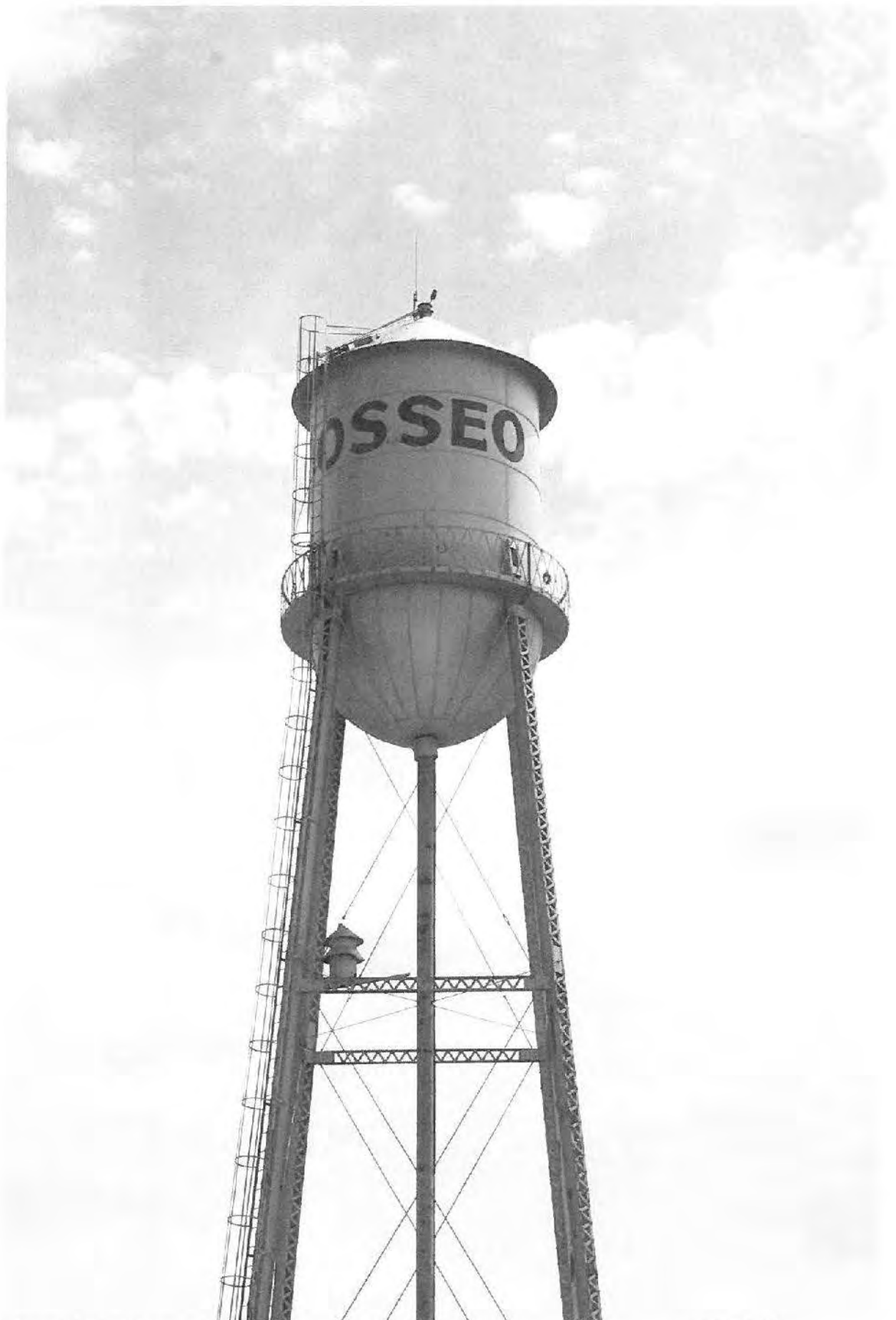
OsseoWaterTower_0011 View: View of the water tower's 50,000-gallon tank
