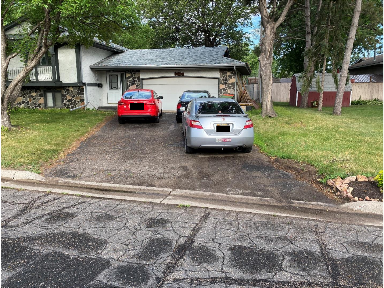
209 9 th Ave NE- ponding.
