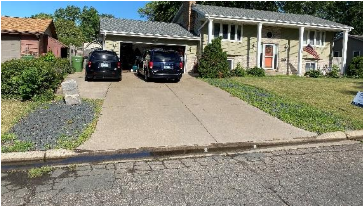
25 8 th Ave NE- ponding.
