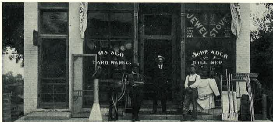
A Hardware store before 1900.
