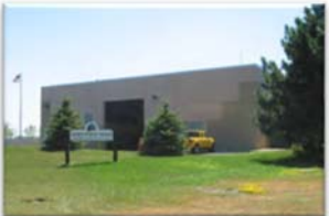
FIGURE 6-2 OSSEO PUBLIC WORKS BUILDING
