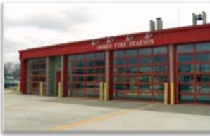
FIGURE 6-5 OSSEO FIRE STATION
