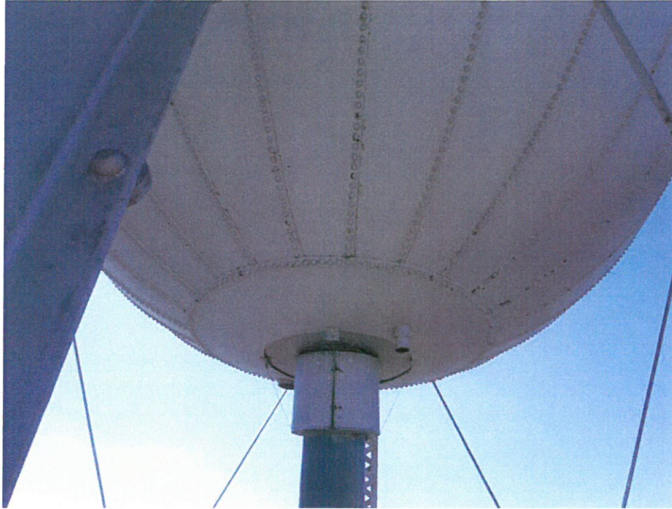
Photo No. 13 Exterior bowl coating conditions
