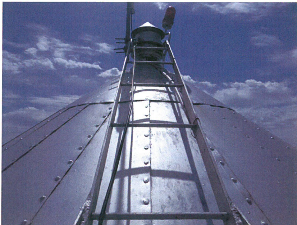
Photo No. 34 Roof finial, obstruction light, and ladder
