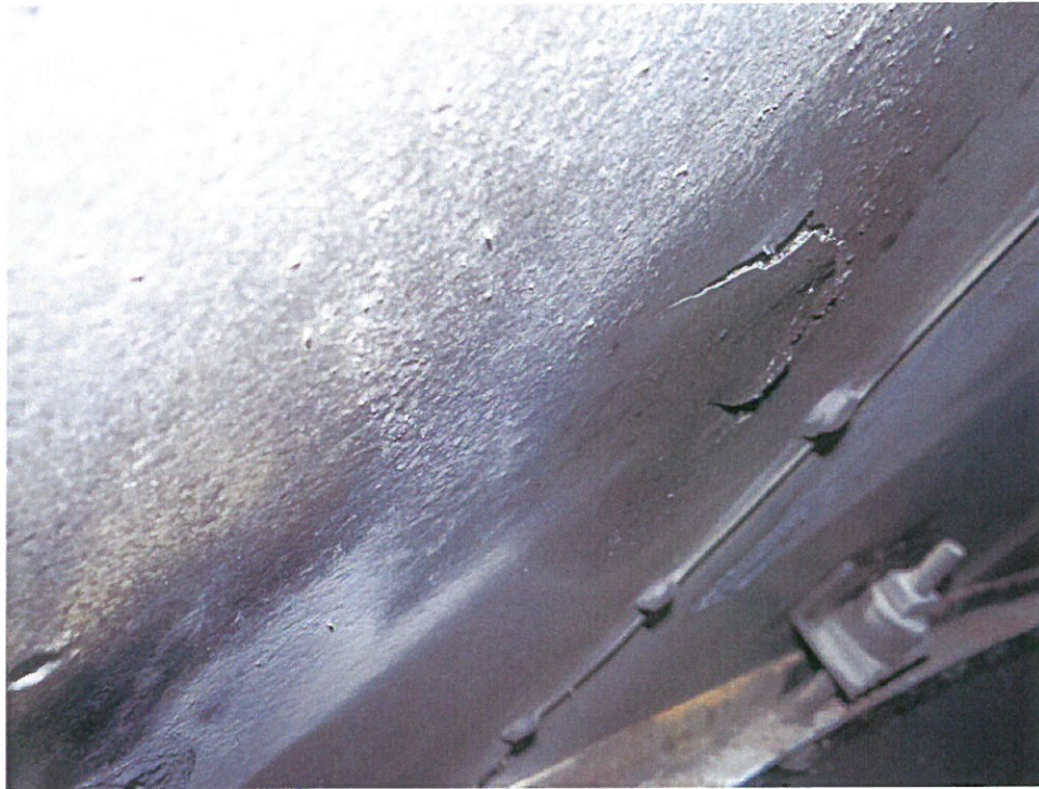
Photo No. 47 Typical conditions on roof – note delaminations
