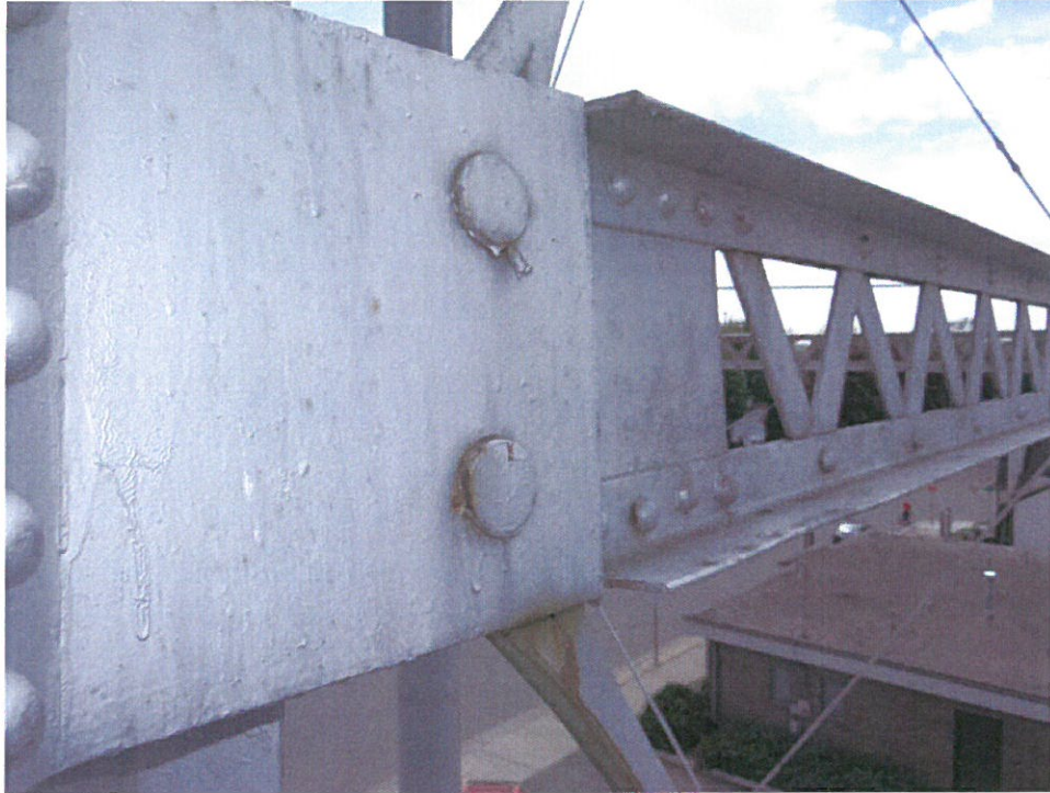
Photo No. 41 Strut truss – note damaged or missing cotter pins at pinned connections
