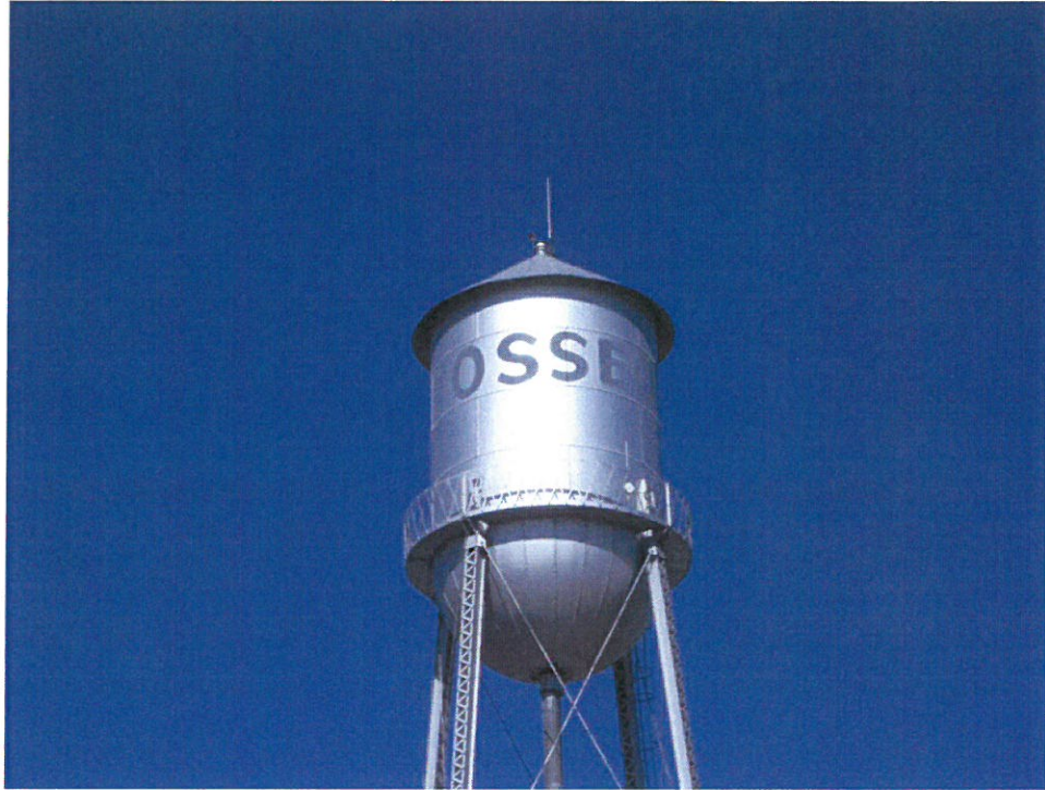
Photo No. 9 Roof as viewed from the ground – note roof ladder attached to finial
