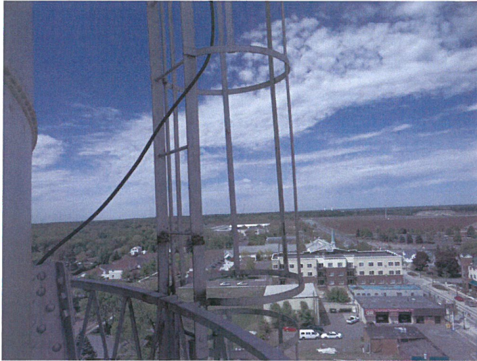
Photo No. 29 Shell ladder following modifications
