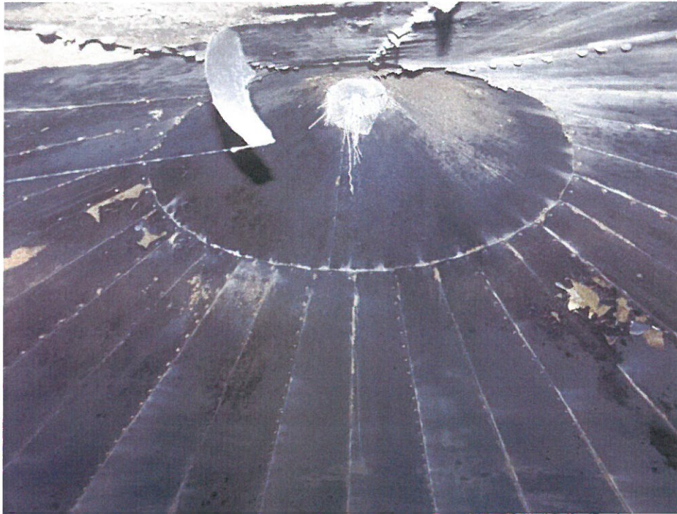
Photo No. 43 Typical conditions on roof – note delaminations
