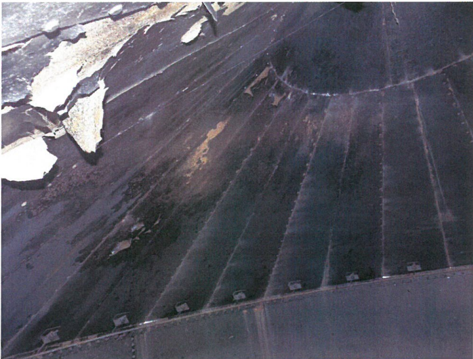
Photo No. 44 Typical conditions on roof – note delaminations
