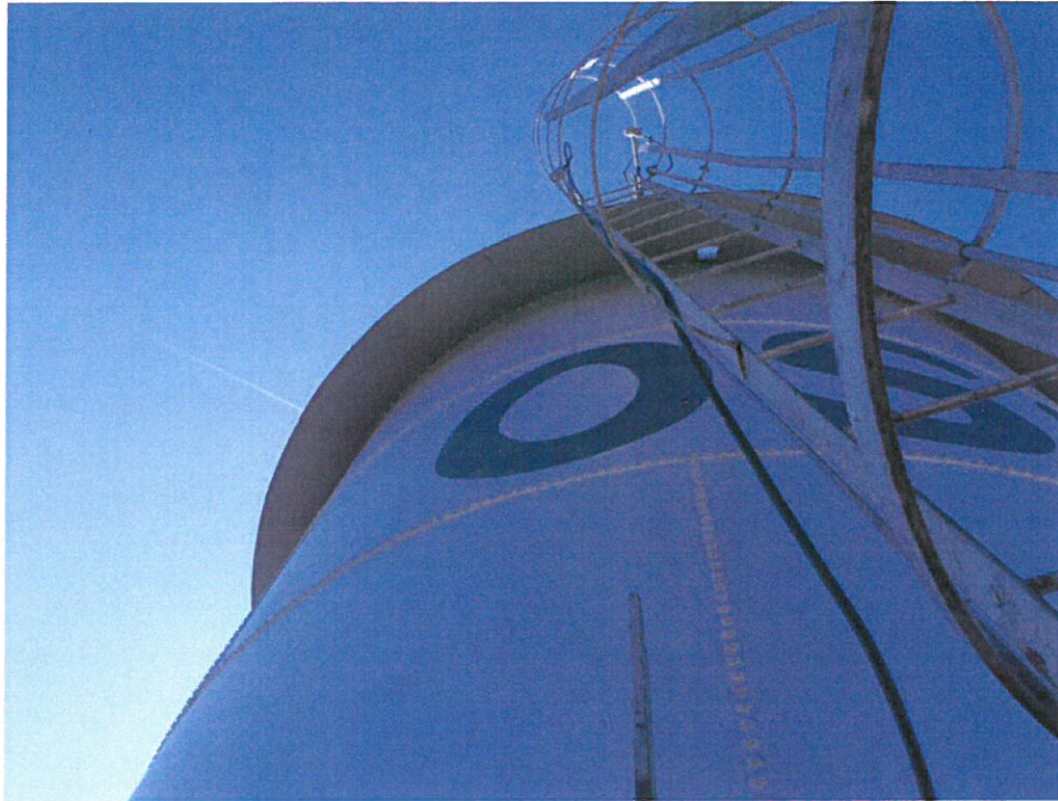
Photo No. 3 Inadequately supported shell to roof ladder
