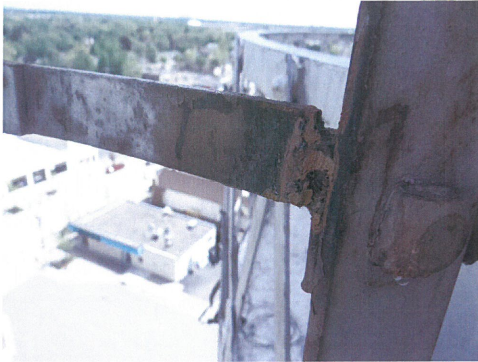
Photo No. 31 Modifications to ladder at balcony
