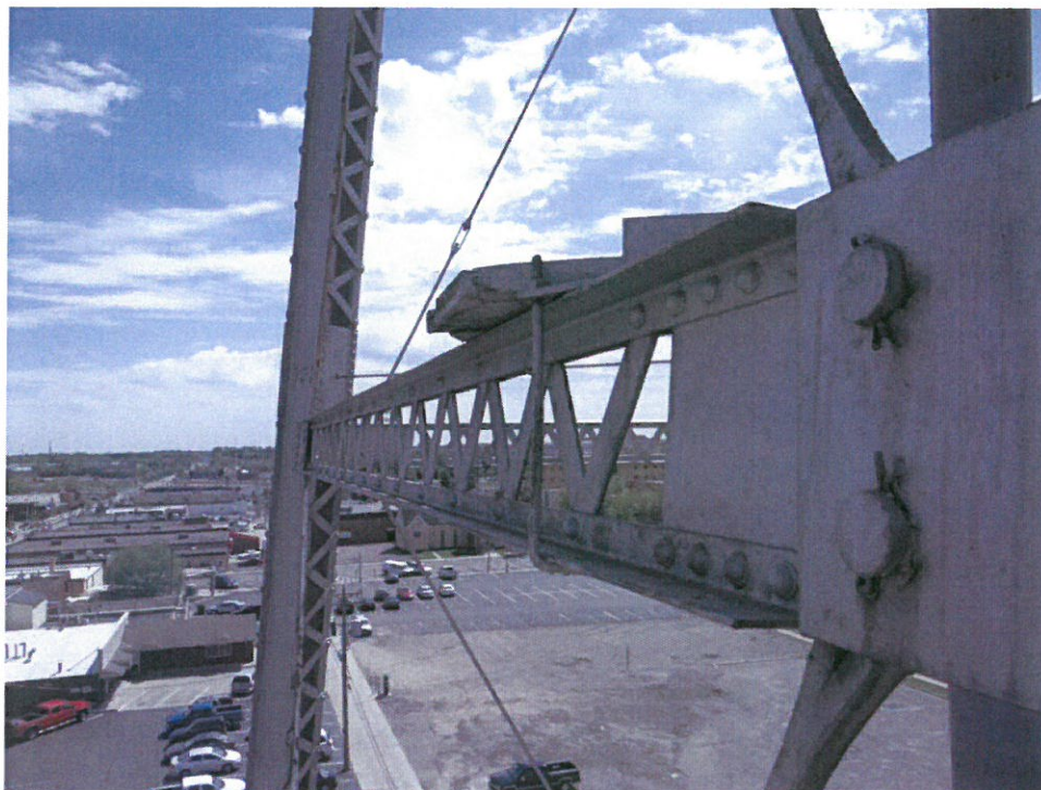
Photo No. 39 Strut truss – note cotter pins at pinned connections
