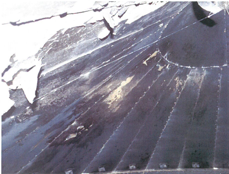
Photo No. 46 Typical conditions on roof – note delaminations
