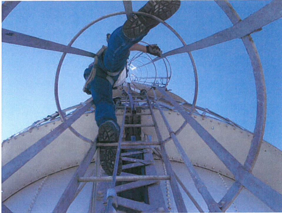
Photo No. 7 Tower access ladder from balcony to roof
