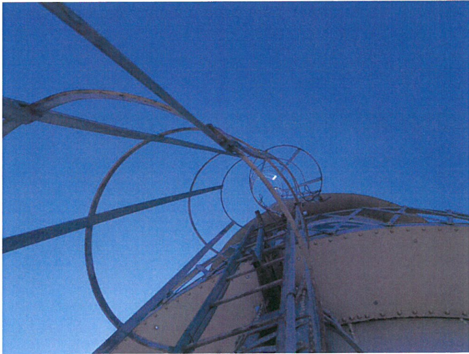
Photo No. 8 Tower access ladder from balcony to roof
