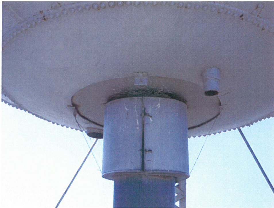
Photo No. 14 Conditions of tower bowl and inlet pipe/expansion joint and frost jacket
