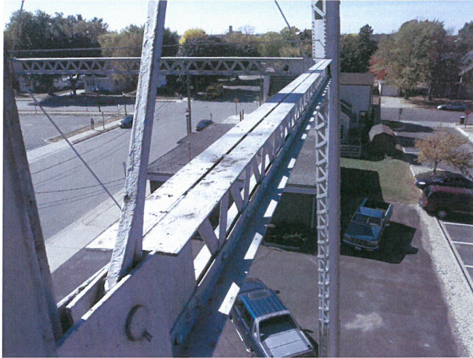
Photo No. 21 Typical exterior coating conditions
