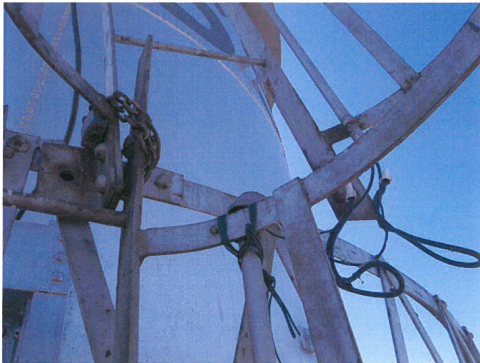
Photo No. 6 Tower access ladder from balcony to roof
