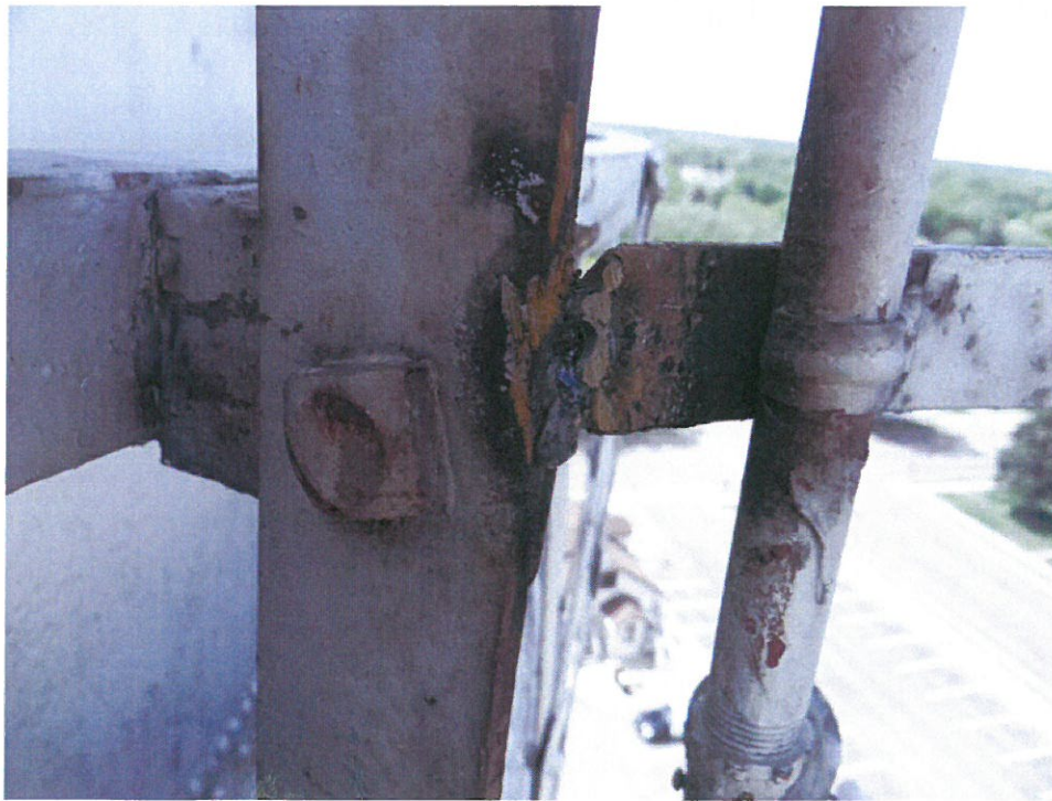
Photo No. 30 Modifications to ladder at balcony
