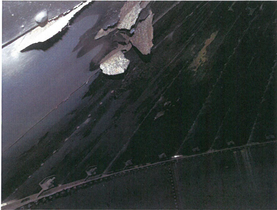
Photo No. 45 Typical conditions on roof – note delaminations
