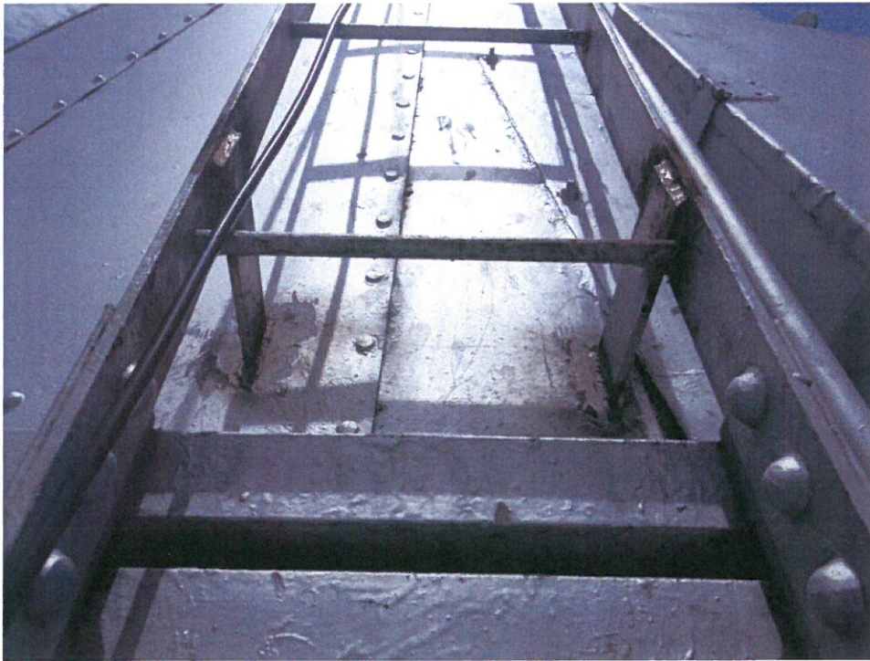
Photo No. 32 Modifications to ladder on roof
